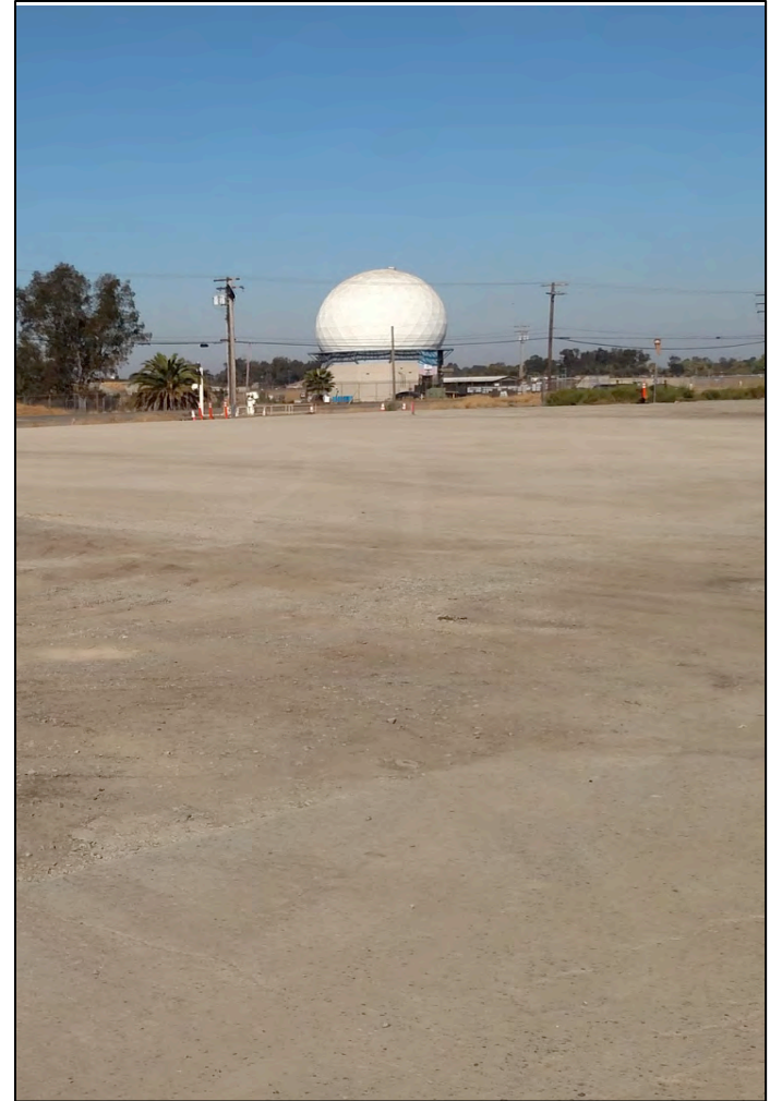
CS043 – Completed backfill.
