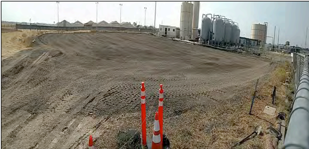
PRL020 – Completed site backfill.
